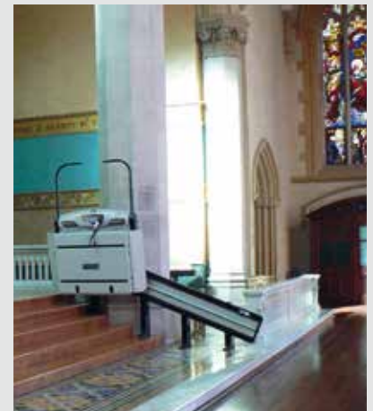
V64 with automated platform folding
